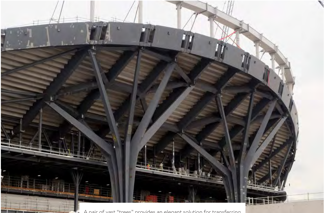
A pair of vast “trees” provides an elegant solution for transferring the huge loads associated with the single-tier South Stand over the sliding pitch below. The main entrance remains uncluttered beneath the spreading “branches”, creating an expansive space for home fans to gather before and after a game.
