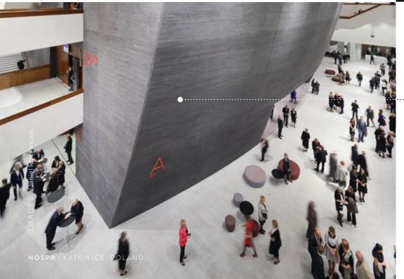
A stand out structure feature is the extremely impressive spherical wall which towers over the atrium. This very complicated shape was only made possible by a series of complex engineering solutions. These included building the wall in several stages, each separated by hollow cross-section elements in order to control cracking of the concrete, whilst keep it hidden at the same time. Even the special concrete mixture itself was developed by BuroHappold in collaboration with the contractor.
