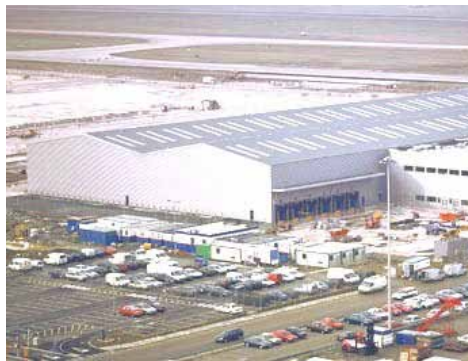
Fedex New Warehouse, Stansted Airport 2000
