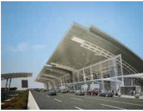
New Doha International Airport, Qatar Ongoing
